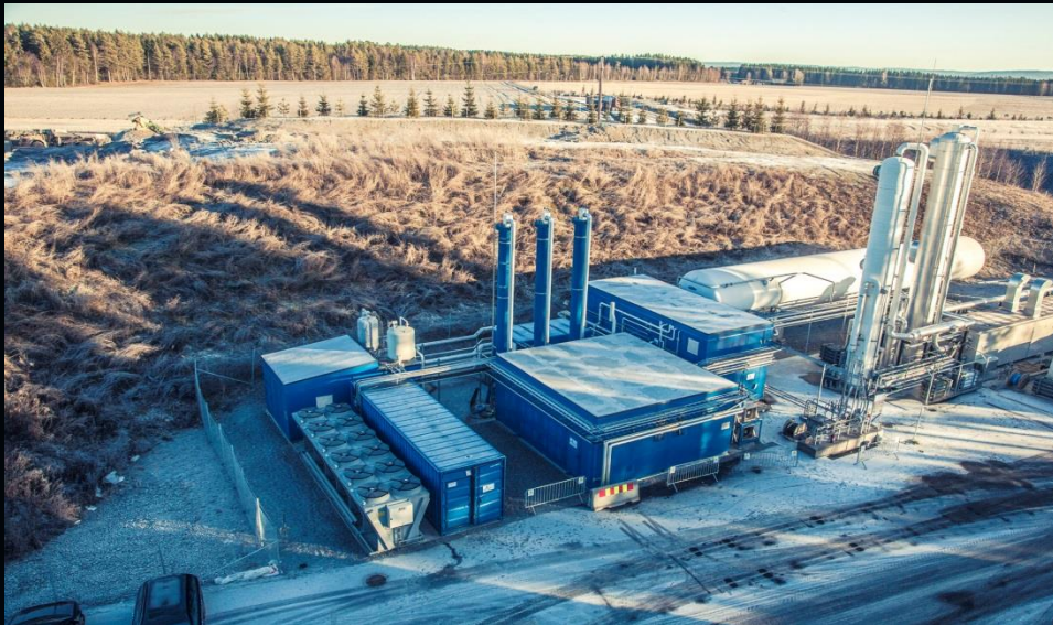
Enclosed waste water treatment plants are environmentally safe and clean
