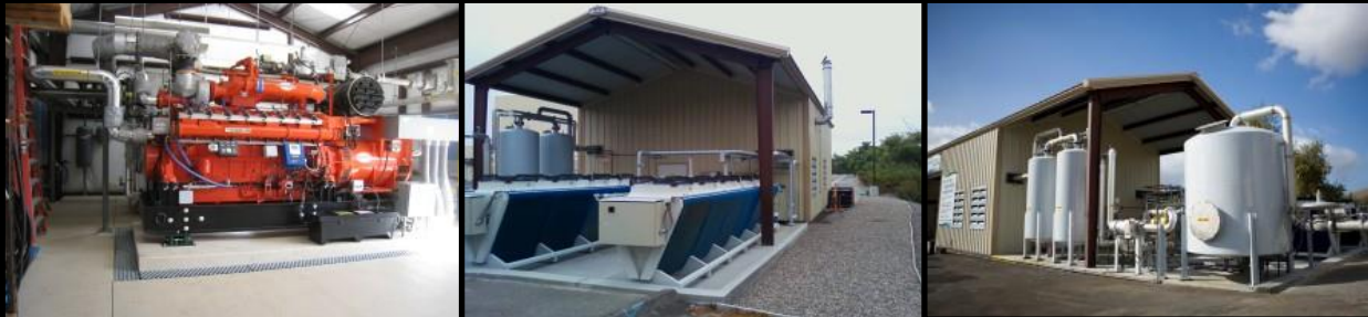
1.5 MW Biogas Renewable Cogen Plant for a Wastewater Treatment Plant - City of Oceanside, CA
