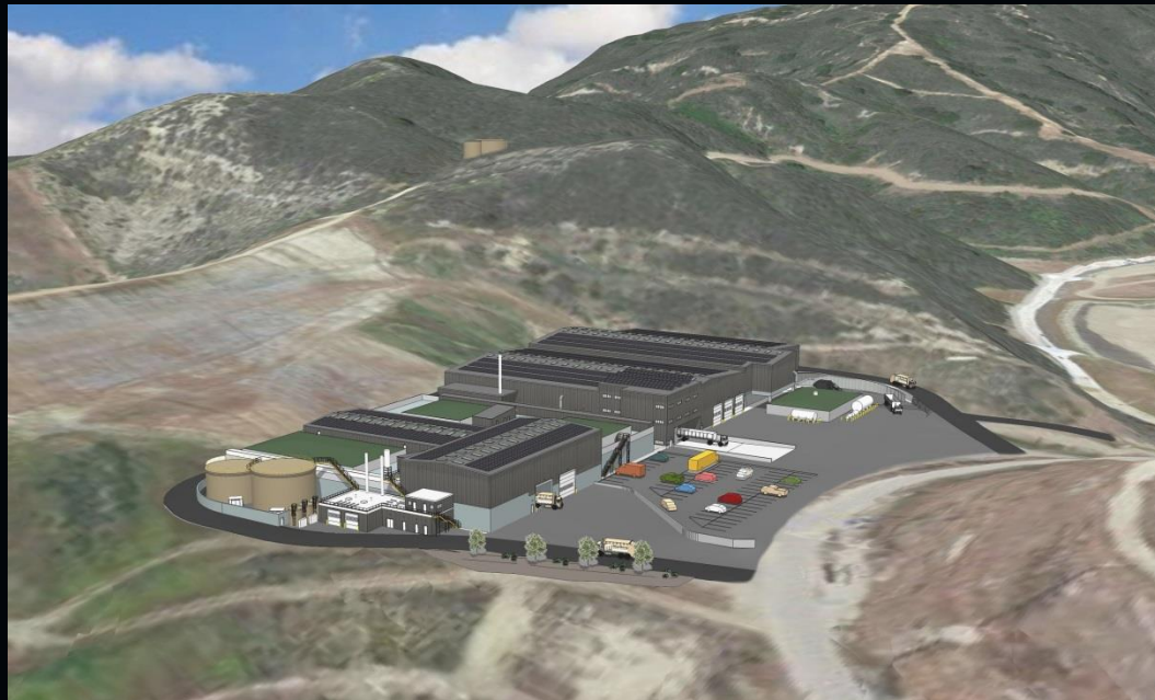
Tajiguas CA, Biogas facility, by Bekon, will process 75,000 tons of biomass a year.
