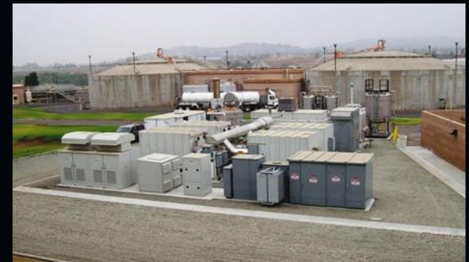
1.2 MW DFC1500 fuel cell power plant
