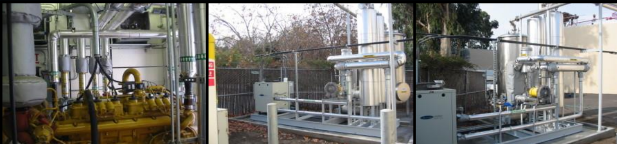
200 kW Digester Gas-Fired Cogen Plant for a Wastewater Treatment Plant - Burlingame, CA
