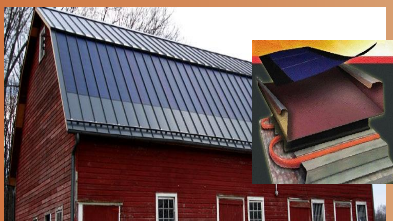
Combined Solar PV and Thermal Systems generate power, provide hot water for ag production and reduce building thermal loads.
