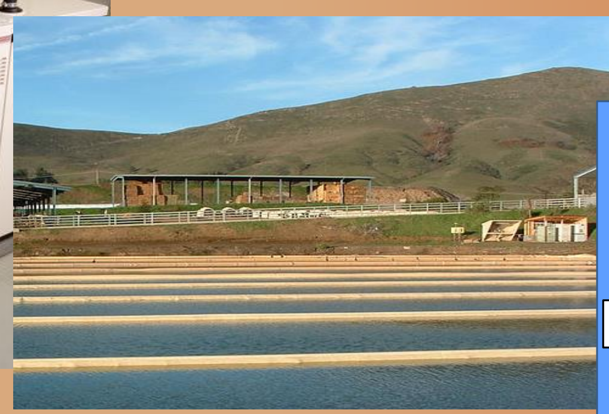
Anaerobic lagoon and 25kW Bio-Gas Generator at the Cal Poly Dairy
